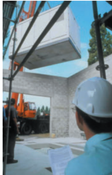
Installation of a fuel cell ONSI in Chelles, France. Gaz de France.
