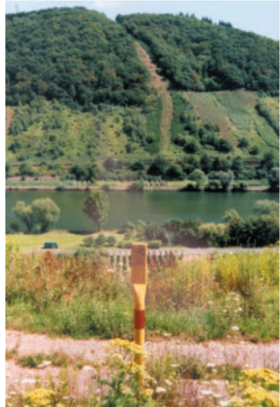
Underground natural gas pipeline crossing the river Mosel.
